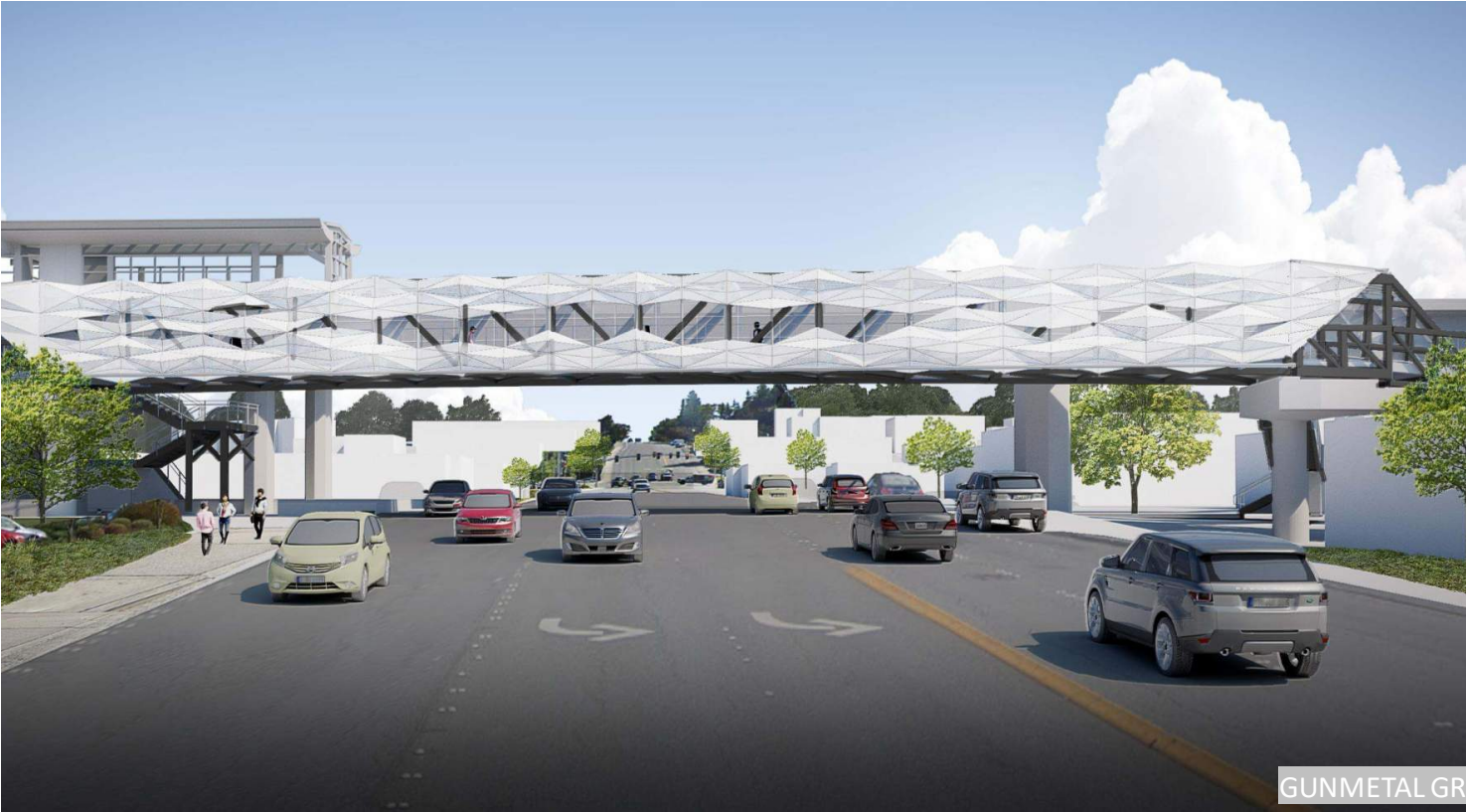
Bridge as viewed from NE 8th St.
